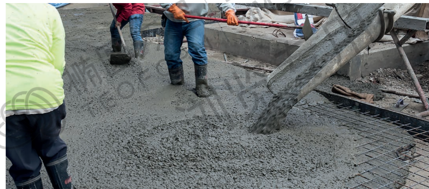
Above: BIM needs structure and guidance - like concrete being poured into a slab.
